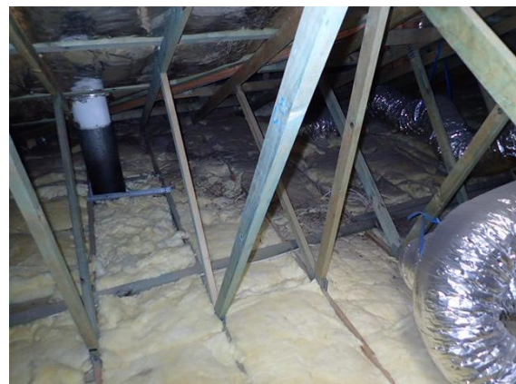
Yellow batts in place
