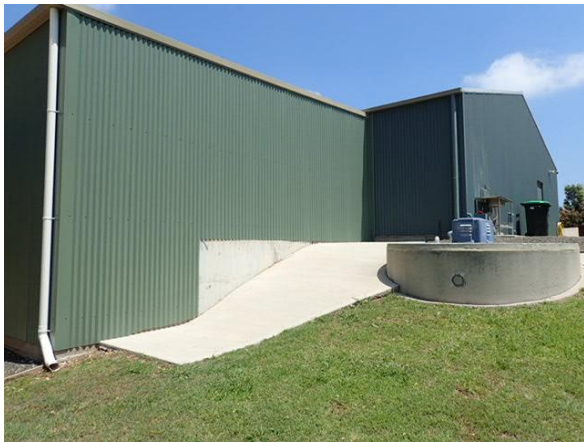
Metal garages in good order
