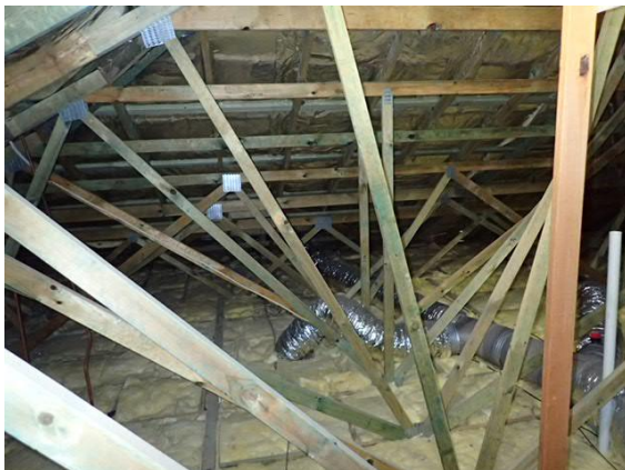
Treated pine roof frame and sarking blanket in place
